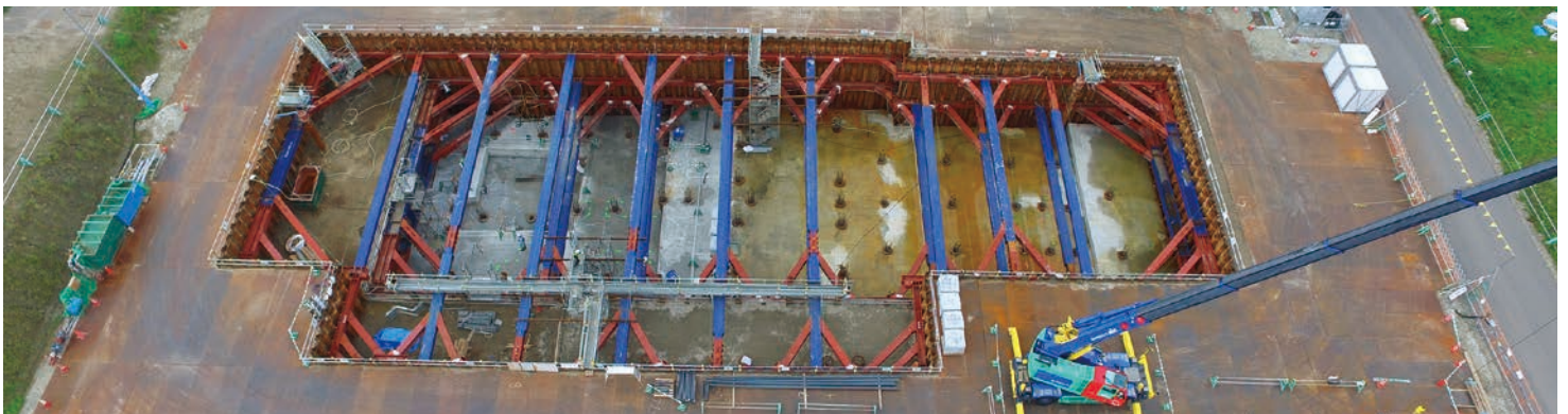
Earth-retaining construction【Hirose twin beam】
