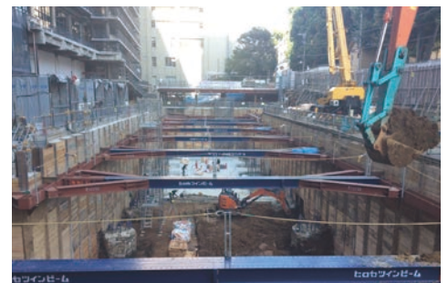
Earth-retaining construction【Hirose twin beam】
