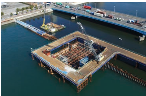
Temporary jetty for construction【G-pilled jetties】
